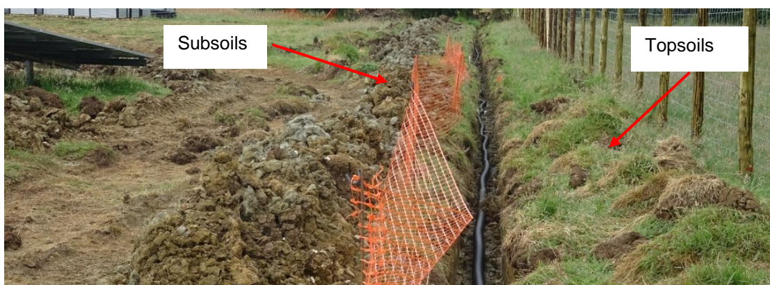
Insert 12: Subsoils Dug out of the Trench
