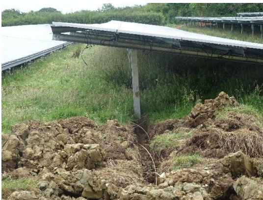
Photos 23 and 24: Cabling Channels During Cable Installation
