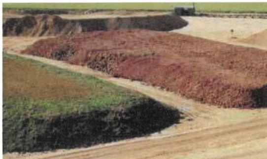
Clearly defined stockpiling of different soil materials
