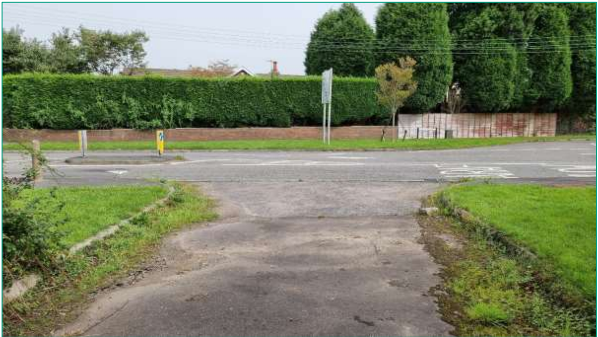
Image 6 - View east across B4620 from existing access.
