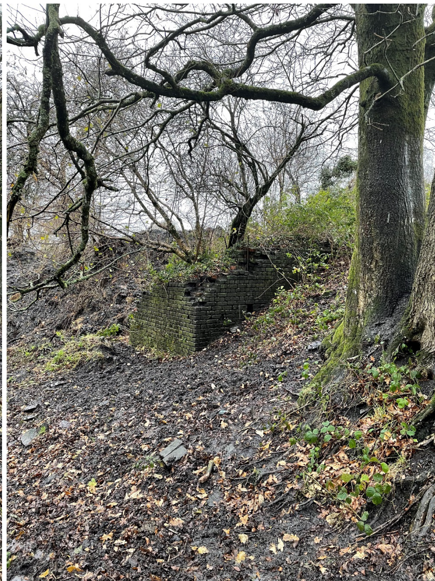
11. Brick structure on east side of pile/drift, viewed from the east
