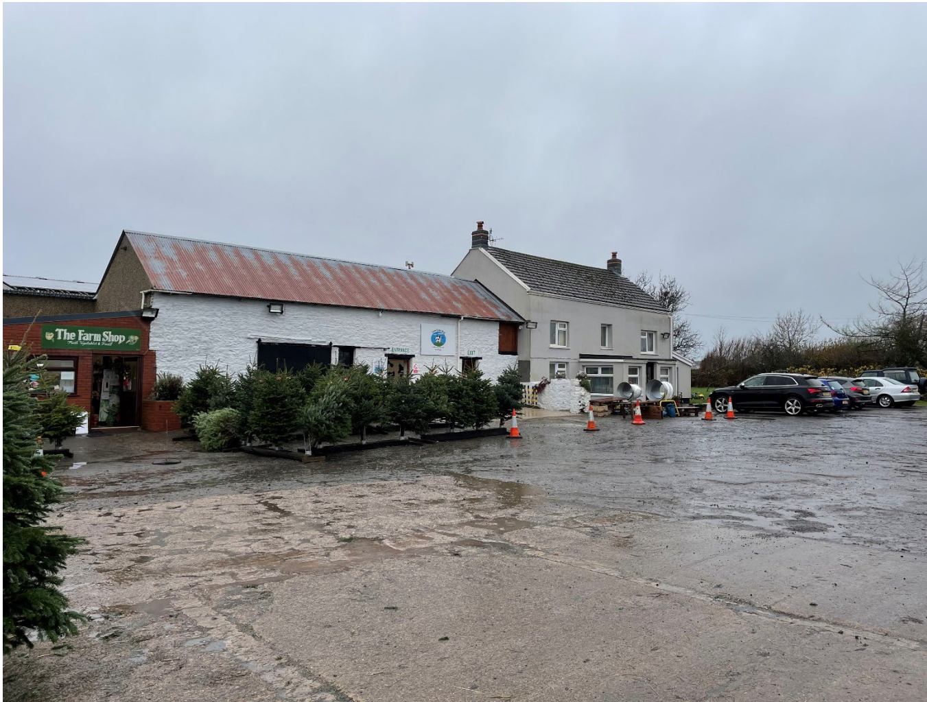
1. East-south-east facing elevation of the farmhouse and its attached barn
