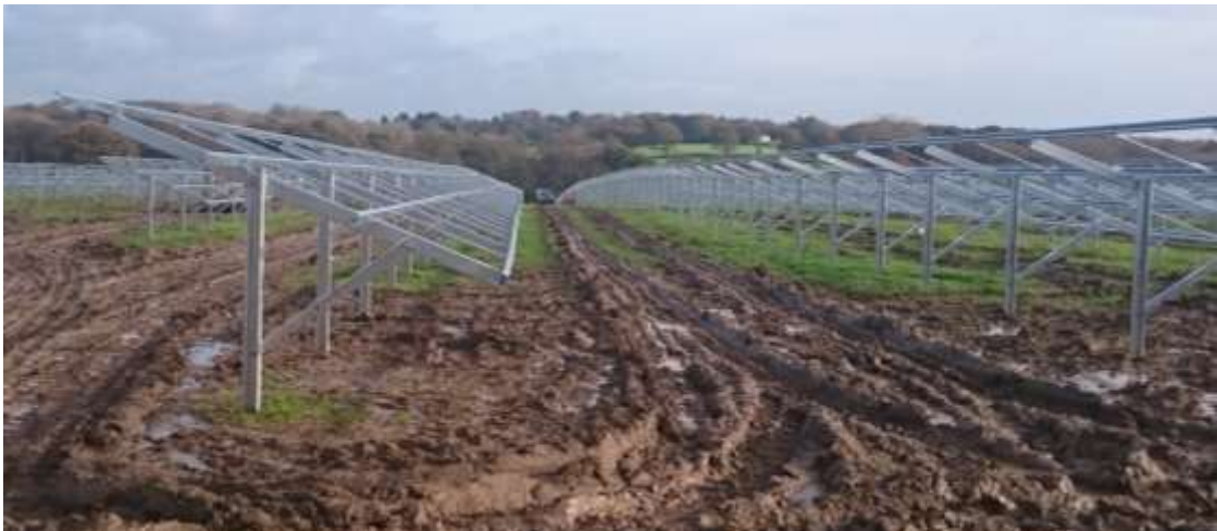
Inserts 1 and 2: Inter-row Ground Restoration
