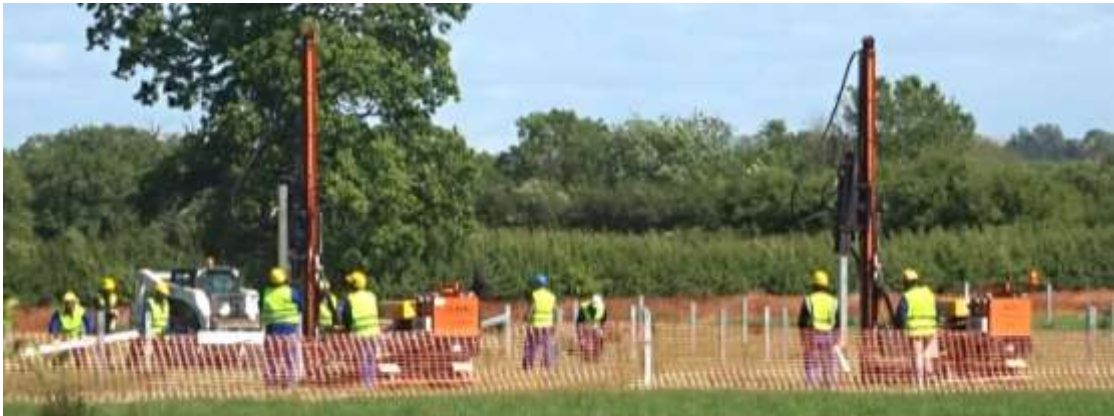
Photo 17: Legs Being Installed
