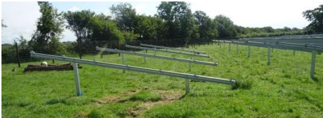
Photos 18 and 19: Legs Installed (this at Bentham Farm, Purton)
