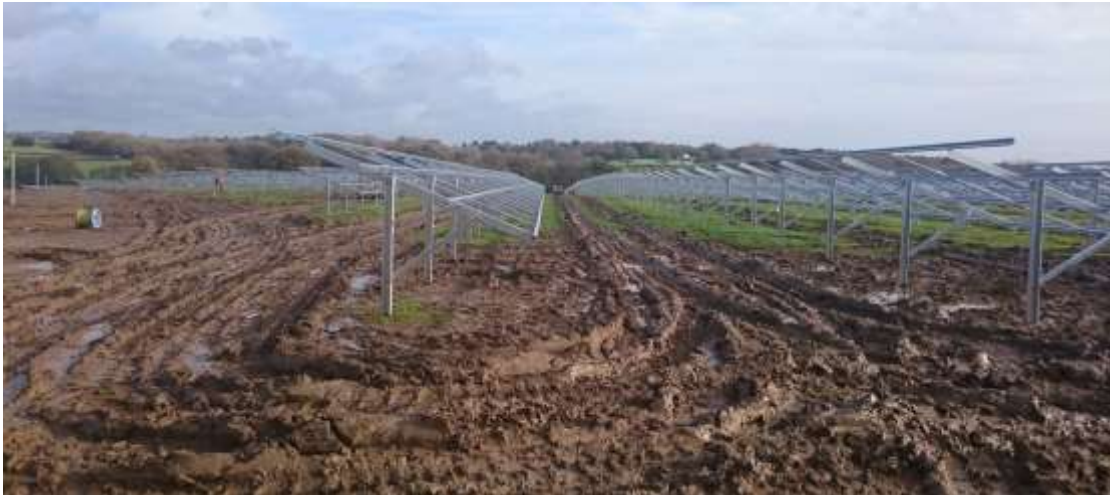
Photos 21 and 22: Panels Installed in Poorer Conditions
