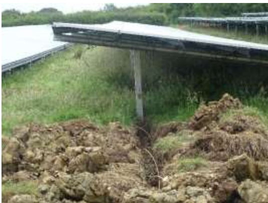
Photos 23 and 24: Cabling Channels During Cable Installation
