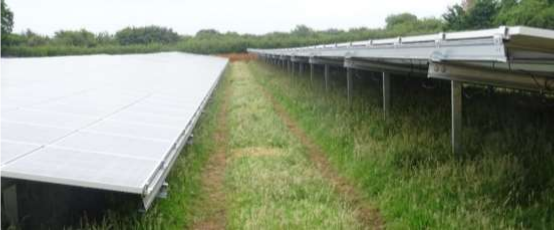
Photo 20: After Panels Bolted-on
