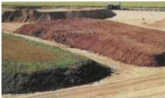
Clearly defined stockpiling of different soil materials
