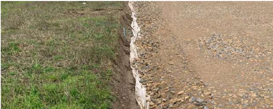
Photo 28: Creation of Access Track (detail)
